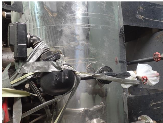
Figure D.36.28 Series 150SJ Low Water Cut-Off/Pump Generator
