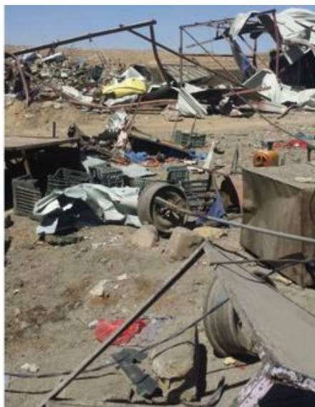
Figure D.58.2 Post strike damage in outer night market area 95
