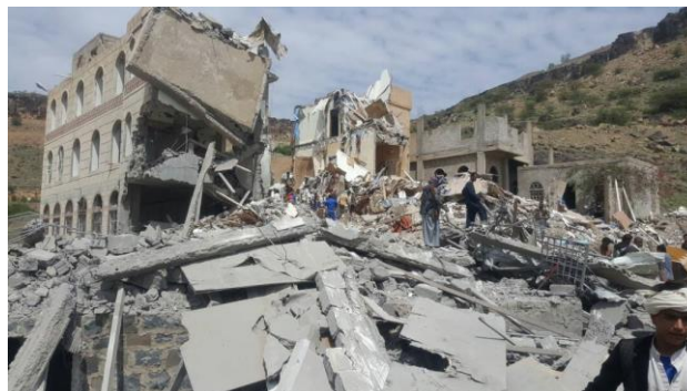
Figure B.58.4 Post-blast damage
