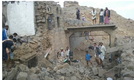
Figure C.58.5 Damage to al-Maqadhi houses
