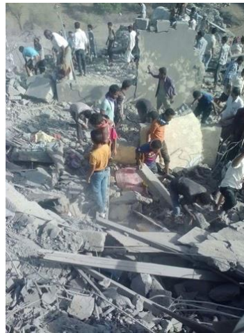
Figure E.60.2 Post blast damage
