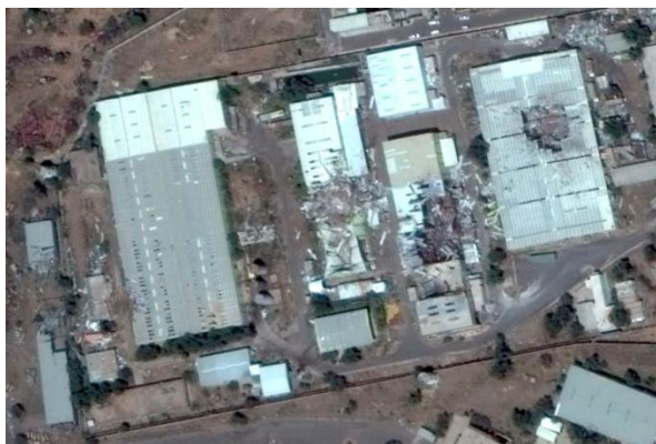
Figure A.60.4 Second strike damage (Post August 2016)
