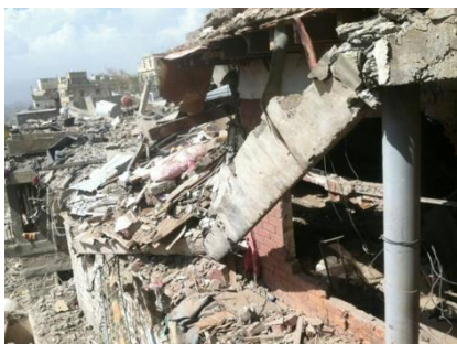
Figure 64.1 Example of damage to house in Ta'izz caused by indiscriminate use of EO
